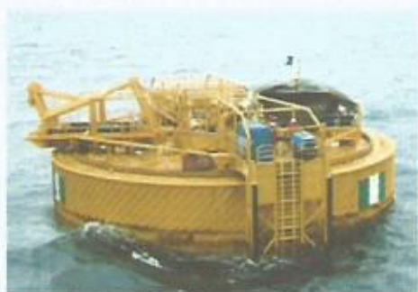
Gambar 2. Single Point Mooring
