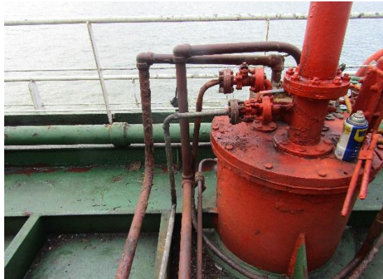
(Sumber : Lewmar (2017). Windlass and anchor operation basic safety ) Gambar 2.14 Pompa Hydraulic
