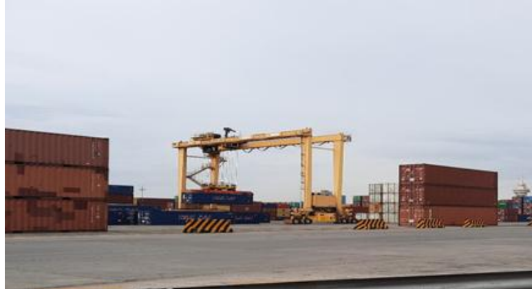
Gambar 1. RTG Crane ( Ruber tyred Gantry )
