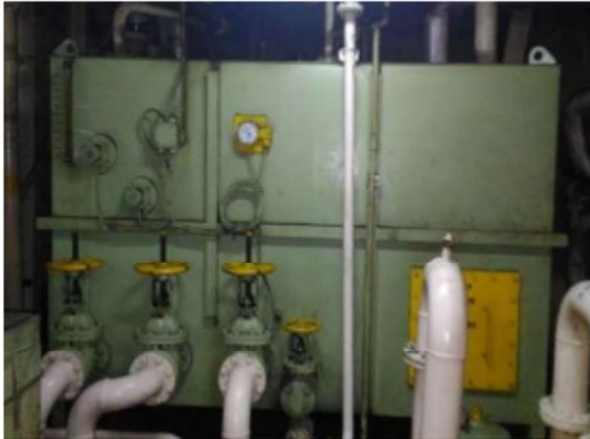
Gambar 2.3 *Hydraulic Oil Tank*
