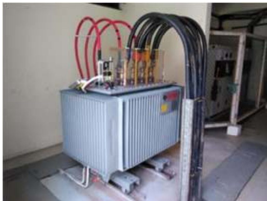
Gambar 6. Trafo Distribusi
