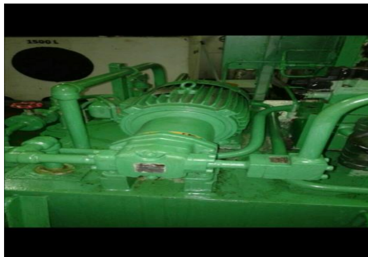
Gambar 8 Hydraulic Oil (HO) Pump
