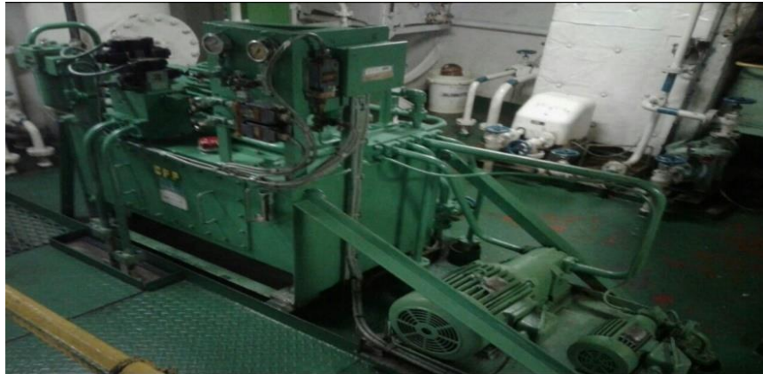
Gambar 9 Komponen Hydraulic Power Pack Sumber: http://Hydrolikmarine.com/auxiliary-engine.html
