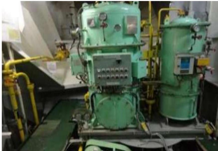
Gambar 1. Oil Water Separator (OWS).
