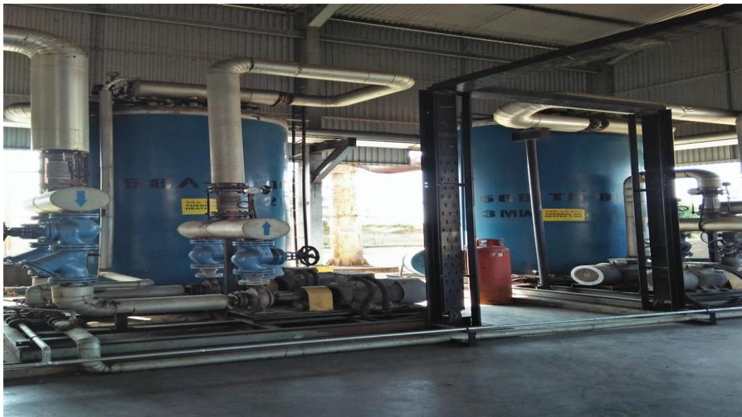
**Gambar 1** *Thermal oil heater*
