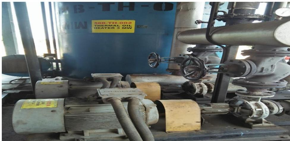
**Gambar 12** Pompa sirkulasi (*Circulating Pump*)
