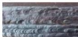
Gambar 10. Unacceptable Weld Profiles
