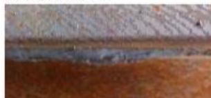
Gambar 8. Excessive Concavity Weld
