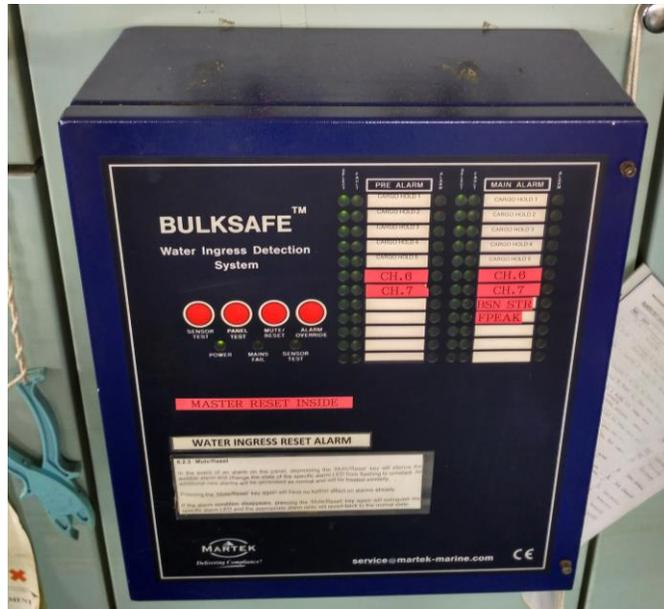
Gambar 2.2. PANEL WATER INGRESS MONITORING SYSTEM
