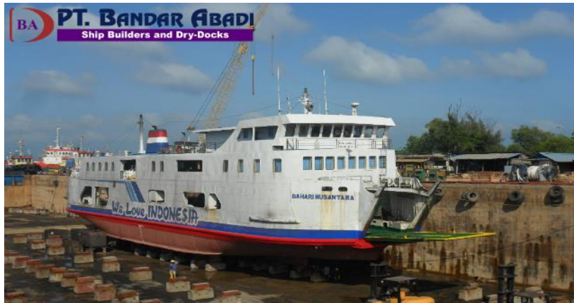
Gambar 2.2 Repair dock shipyard
