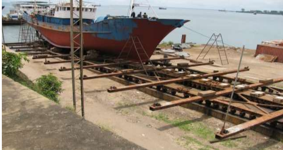
Gambar 4 Dok Tarik ( Slipway Dock ) Sumber: Dokumen Asli
