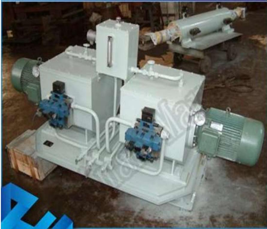
Gambar1 Electro Hidrolik Steering Gear.
