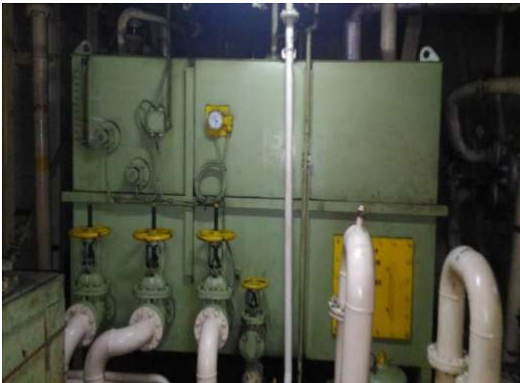
Gambar 2.1 Hydraulic Oil Tank
