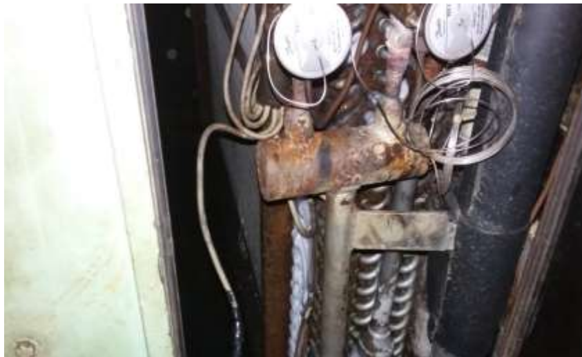
Gambar 5. Evaporator
