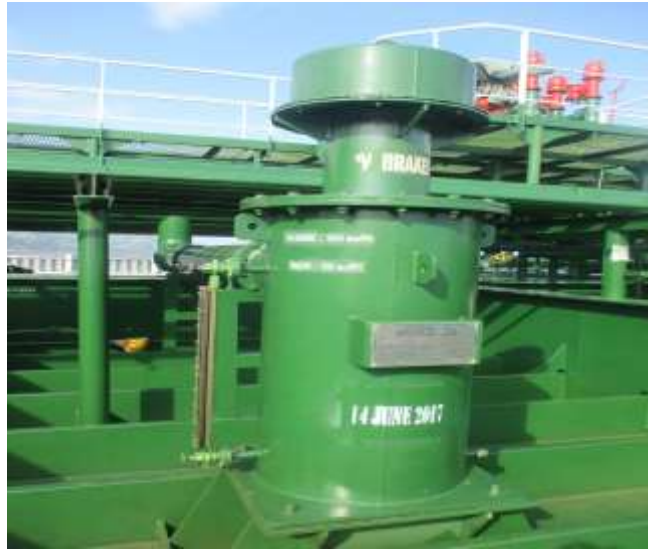
Gambar 12. Pressure Vacuum Breaker
