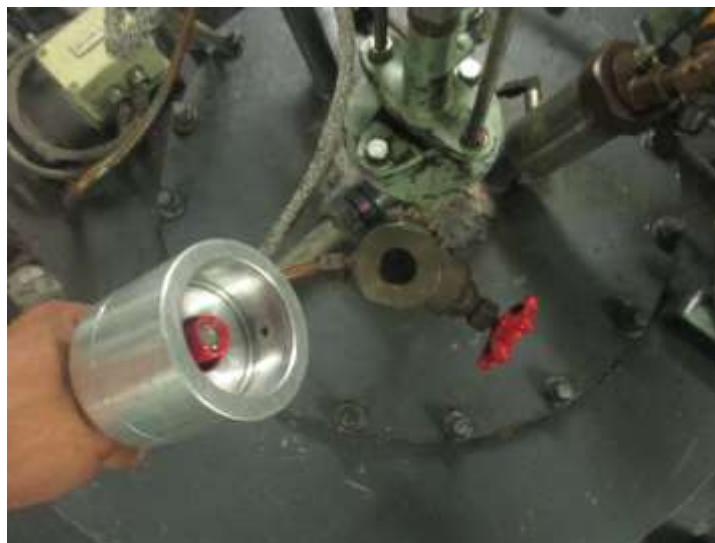
Gambar 17. Flame Eye Sensor
