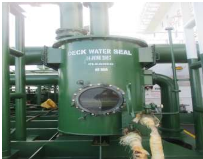
Gambar 8. Deck Water Seal Unit
