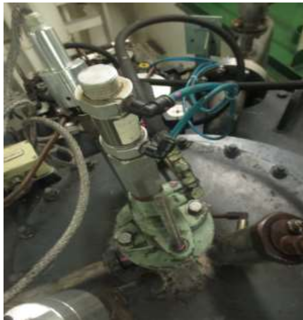
Gambar 13. Main Burner
