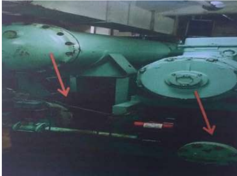
Gambar 5. Evaporator dan Oil Separator (Sumber: KM. SIMORE)
