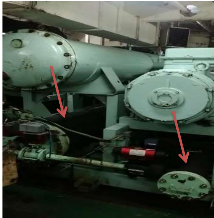
Gambar 3. Evaporator dan Oil Separator
