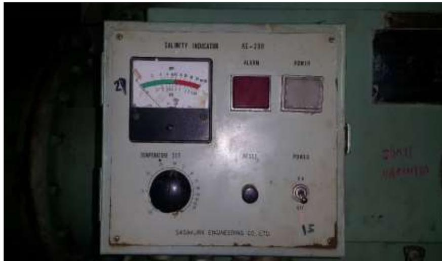
Gambar 8 Salinometer / *Salinity Indicator*
