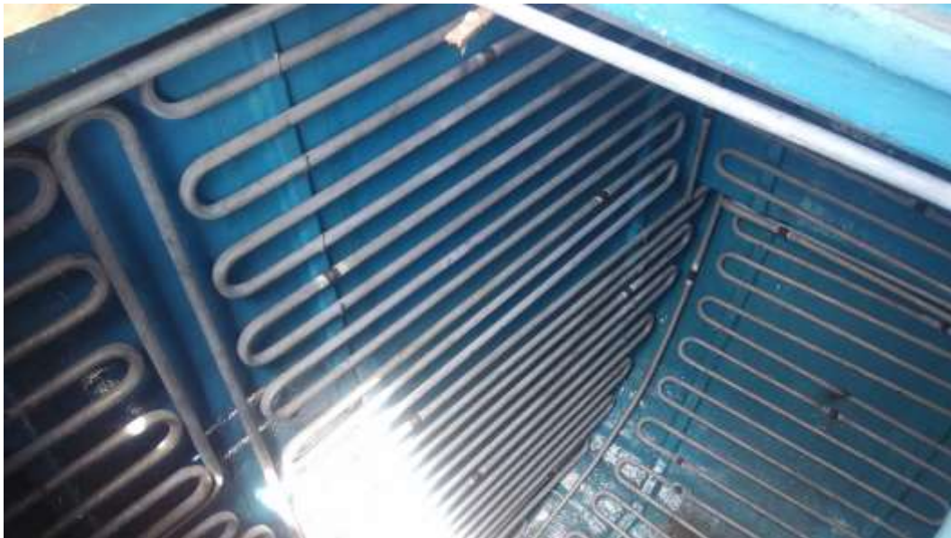
Gambar 1.8. Penampang Evaporator didalam Palka
