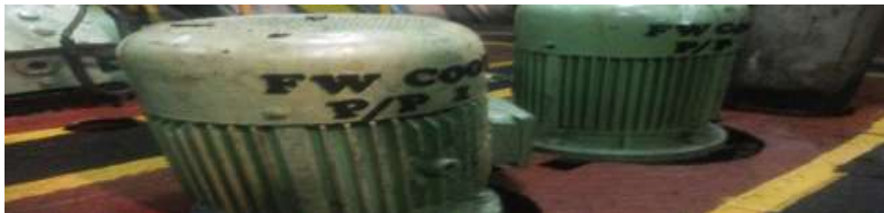
Gambar 3. : Pompa Fresh Water (Sumber : Nurdianto, gambar pompa FW.2001)
