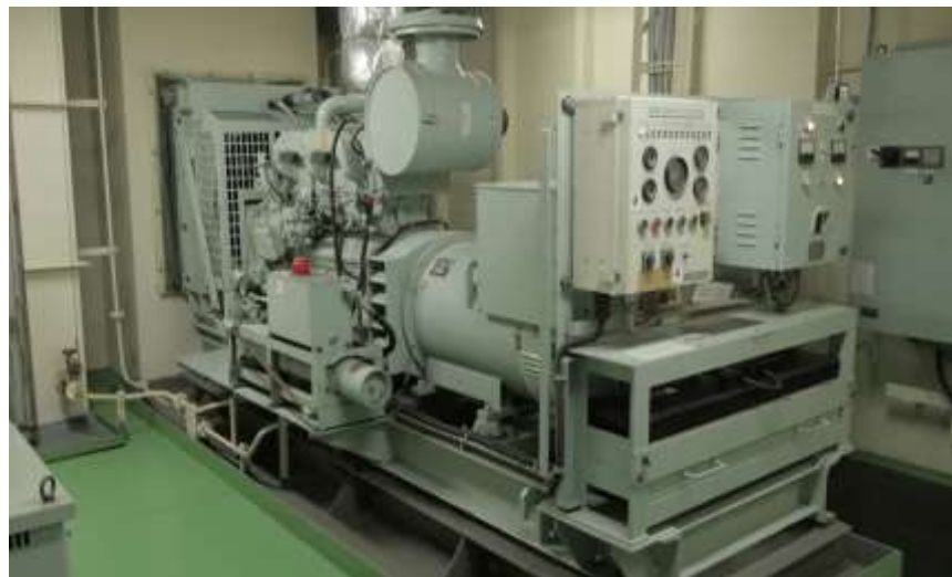
Gambar 1 Diesel Generator (John D. Mc Donald 2007 Electric Power Substations Engineering , CRC Press : London)
