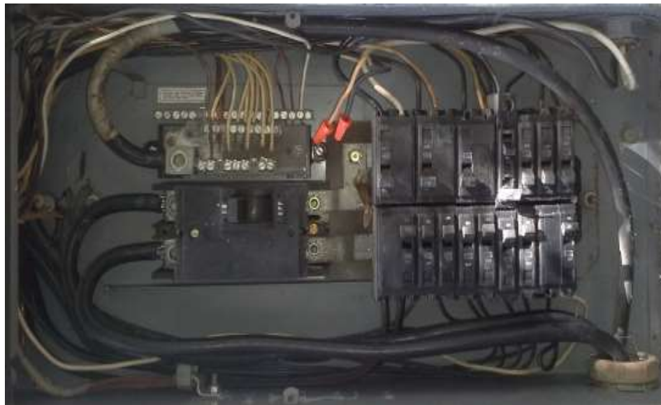
Gambar 15 Rangkaian Dead Front Panel
