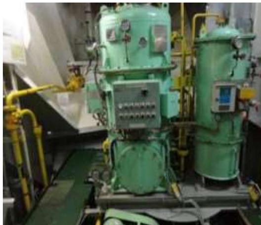
*Gambar 1 Oil Water Separator*
