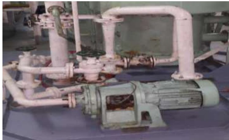
Gambar 6 Ejector Pump
