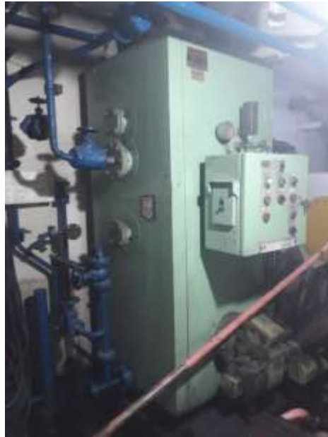
Gambar 1. Boiler MV. Sumber Cahaya
