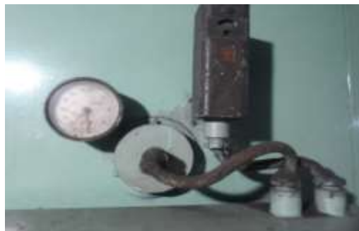
Gambar 7. Safety valve MV. Sumber Cahaya
